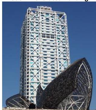
Modern Ventilated Building
